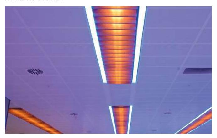
The Tacer Hook-on Series are suspended ceiling solutions where special carrier systems interlock using a hook-and-clip method, allowing for an invisible ceiling surface and the flexibility to go beyond standard dimensions. These systems are typically produced in 600x600 mm sizes and can also be custom-made according to project-specific dimensions.
