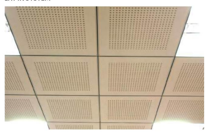
The Tacer Acoustic Gypsum Tile Lay-in Board Suspended series is a ceiling system supported by special carrier systems, which allows for height differences to be highlighted and is suitable for grid planning on the ceiling. Tacer Acoustic Gypsum Board suspended systems are panels that can be planned in standard or custom sizes, designed to support the project and space.
