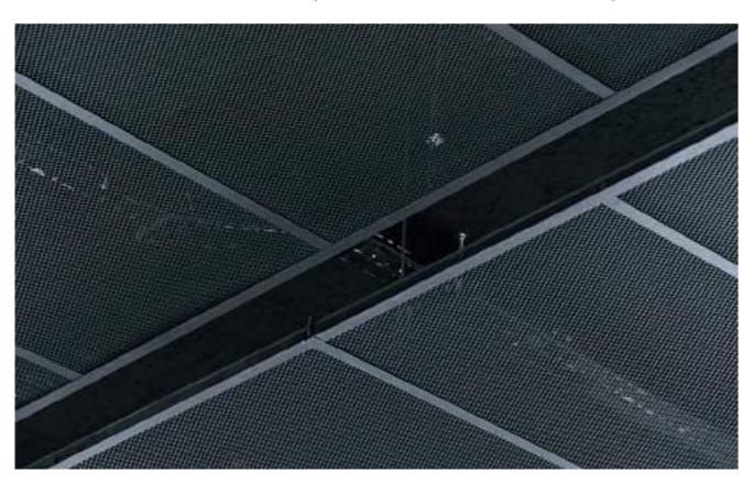
Tacer Diamond metal systems are solutions supported by special carriers with T24 or T15 profiles, which can be produced in standard or custom sizes. Thanks to the characteristics of the carriers, they offer a monolithic and clean appearance, while the pattern and design of the Diamond series add movement to the space. With various painting options and a wide range of materials, they adapt to all kinds of spaces and designs.
