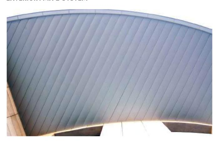
Tacer FMX-2 Systems are suspended ceiling solutions created by claw carrier profiles and specially customized edge-bent profiles, designed primarily for outdoor use. With various size options, the combination of profiles allows for flexible design, enabling them to be used individually or together. It stands out for its resistance to environmental factors, particularly wind load.
