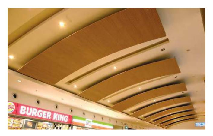
The Wooden Fixed System consists of systems where wooden battens are attached to a steel structure using screws or compressor nails, or created as a tongue-and-groove wall system. In some variants, adhesives can also be used. In tongue-and-groove systems, three types of carrier profiles are used: top, middle, and bottom.
