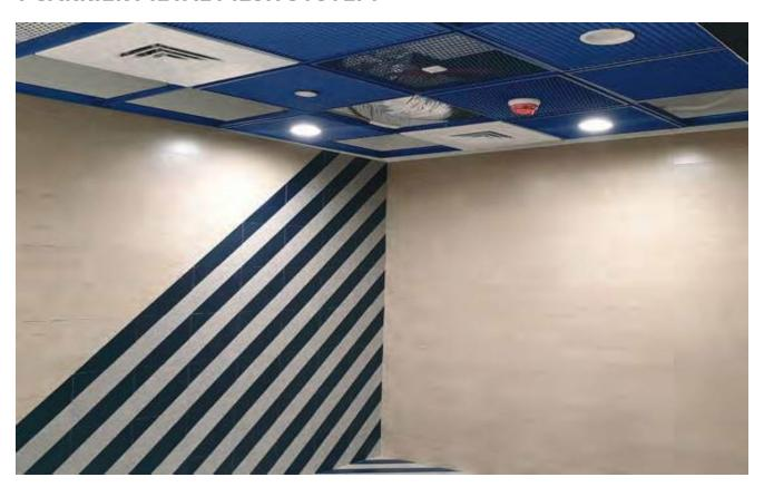
Tacer T Carrier Wide Expanded Metal Systems are suspended ceiling systems produced with special and standard sizes, supported by the edge L profile of T 24 carriers. This system is highly preferred both for its design richness and ease of use. Mesh systems can be designed in desired sizes and orientations, while custom forms can be created according to the user's preference with either pressed or non-pressed options.
