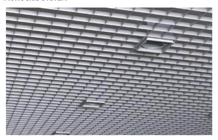
Tacer Monogrid Systems are suspended ceiling solutions created by mounting 600x600 mm or 600x1200 mm monogrid panels onto T24 main carriers. The lightweight panels, available in square and rectangular geometries, allow for modular planning and adapt to different space scales and building modules.
