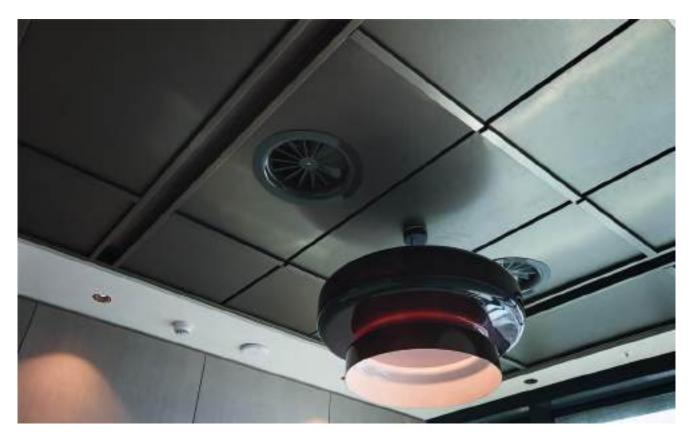
The Tacer Bandraster Series are suspended ceiling solutions that provide compatibility with modular and linear plan modules using C and D section carrier systems. These systems allow for the creation of grid layouts due to the visibility of the carrier profiles on the ceiling surface. With the ability to be produced in custom sizes for different building module scales, these solutions can be easily adapted.
